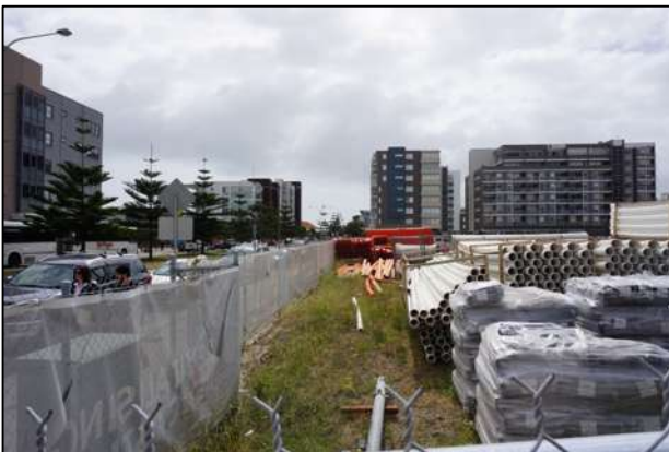
FIGURE 24: INTERIOR OF SITE 1, NORTH. VIEW EAST (SOURCE: CURIO 2018)
