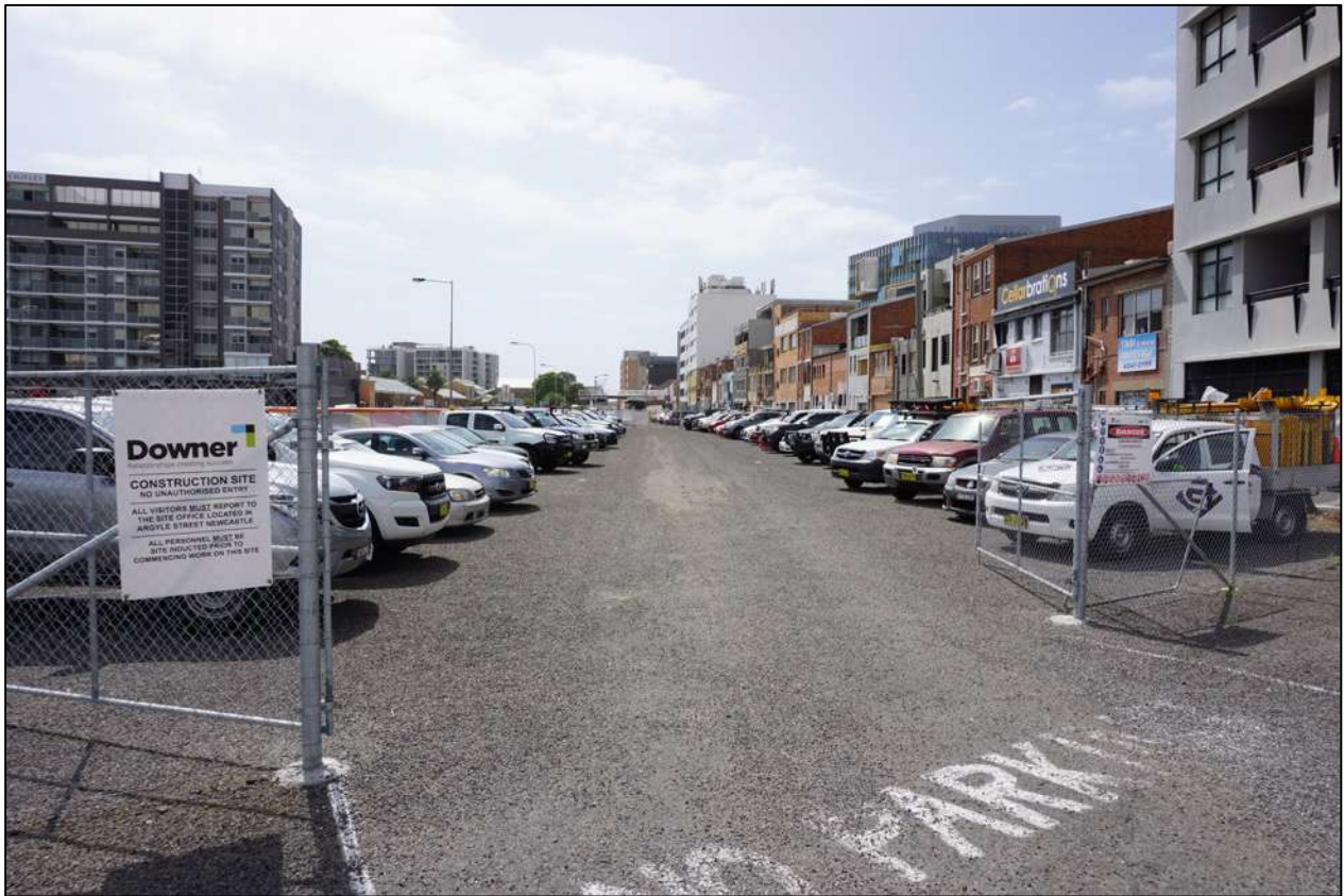
FIGURE 23: VIEW EAST ALONG FORMER RAIL CORRIDOR (SOUTHERN PART OF SITE 2), CURRENTLY USED AS PARKING/CONSTRUCTION STAGING FOR CONSTRUCTION OF LIGHT RAIL (SOURCE: CURIO 2018)
