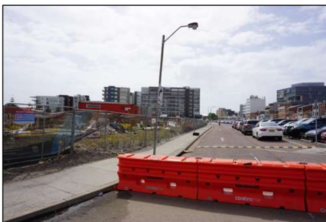
FIGURE 30: VIEW EAST ALONG WRIGHT LANE, BETWEEN SITE 1, AND SITES 2 AND 3 (SOURCE: CURIO 2018)
