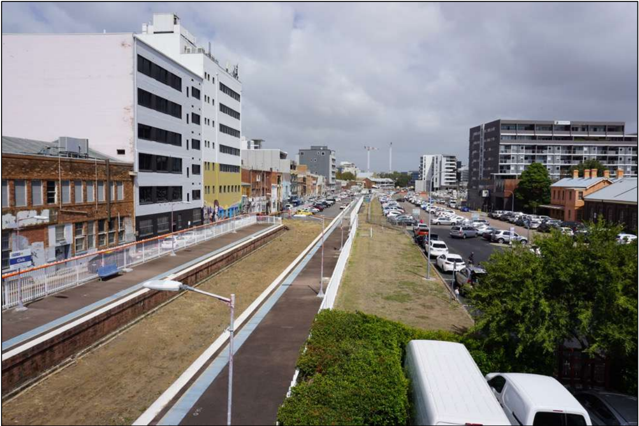
FIGURE 36: VIEW FROM CIVIC STATION, WEST TOWARDS SITES 2 AND 3 (VISIBLE AS CARPARKS IN BACKGROUND) WITH SITE 1 FURTHER IN THE RIGHT BACKGROUND OF IMAGE (SOURCE: CURIO 2018)
